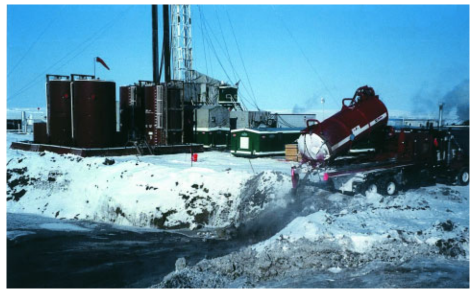
Sump in the Mackenzie Delta. Photo source: Newpark Environmental Services
